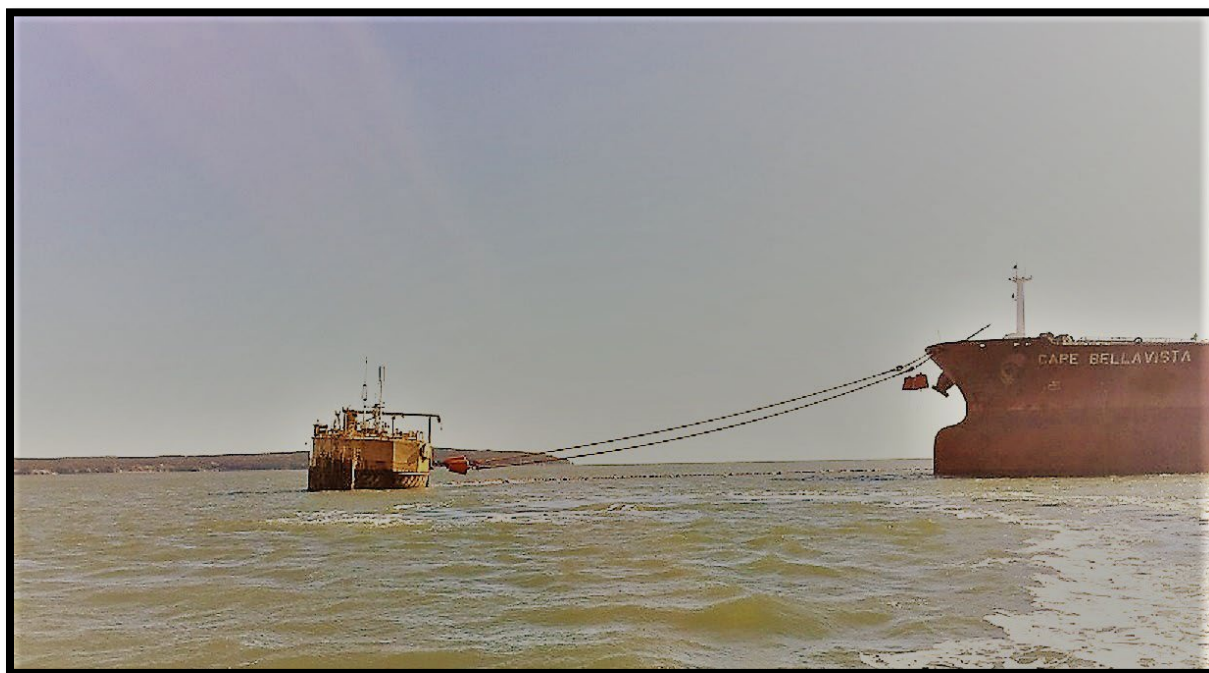
FIGURE 1-8 CALM Buoy with Moored VLCC (Not Project-Specific)
